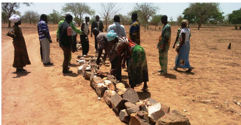
Building rock formations to prevent rainwater runoff and trap fertile soil
